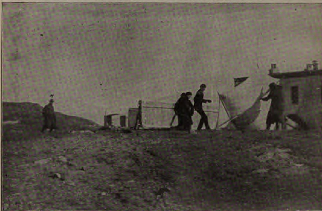
MARCONI'S ASSISTANTS PREPARING TO RAISE THE KITE WHICH SUPPORTED THE RECEIVING WIRE.
